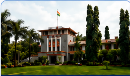
UNIVERSITY ADMIN BUILDING
